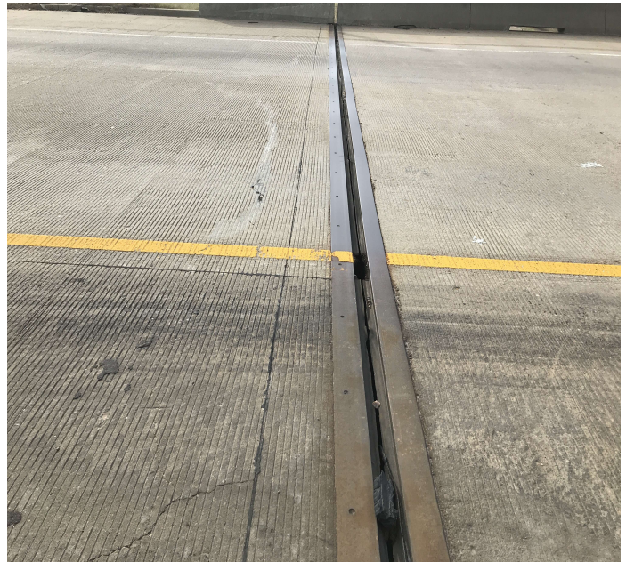
PHOTO 2 Description Abutment #2 joint material is torn full length.
