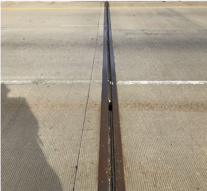
PHOTO 1 Description Abutment #1 joint material has twenty five feet that is torn.
